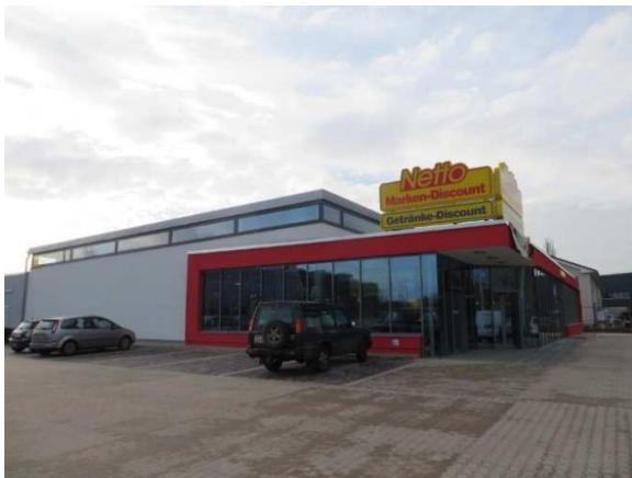
Netto Supermarket – Opening of 1st Passive House Discounter in Hanover, December 2014, Photos © NETTO
