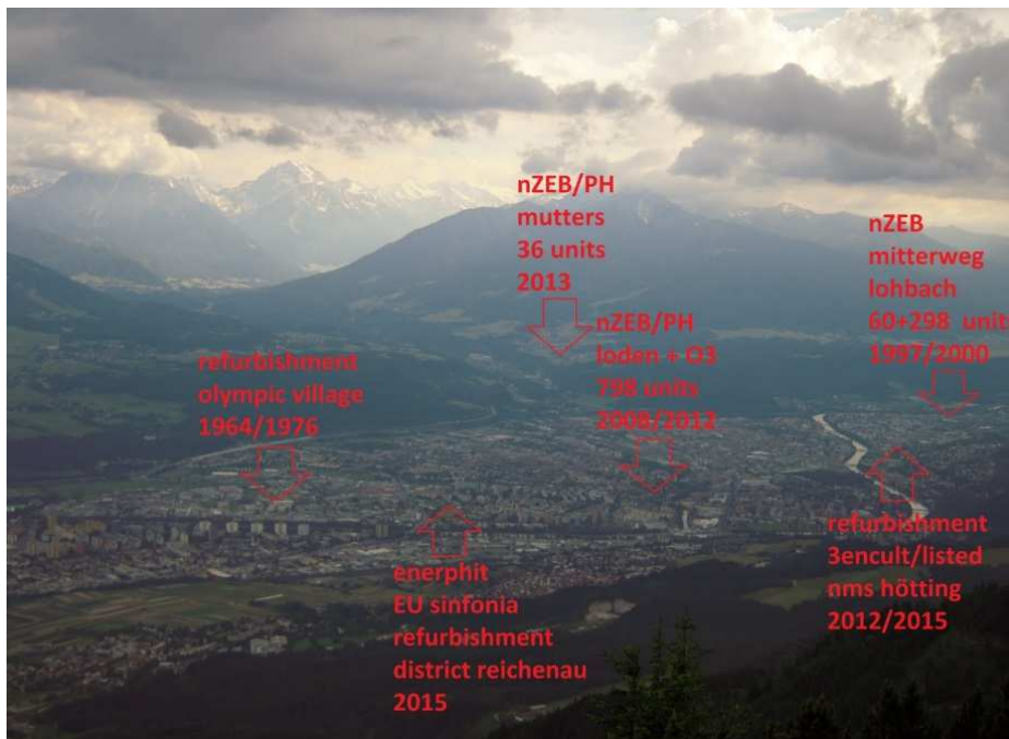
Some examples of NZEB activities and thermal refurbishment within the city of Innsbruck, Photo G.Gaigg © IG Passivhaus Tirol
